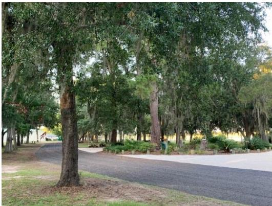
It is composed of 4 inches of reprocessed asphalt, heavily rolled under high pressure. It will hopefully hold up for many years. At the end of its expected long life, it will
